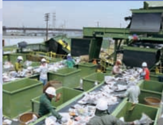
▲ Single Stream Installation City Fibres, USA. Capacity 35 tons per hour.
